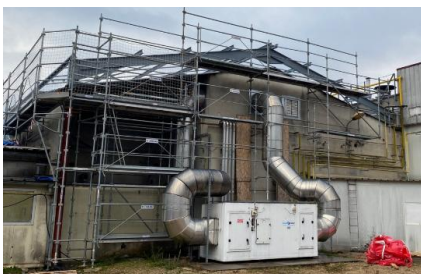
Renforcement de charpente BOLARD – SAINT-AMOUR (39)
